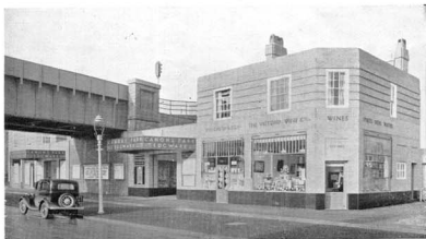
The Metropolitan Railway Station, three minutes from Estate
